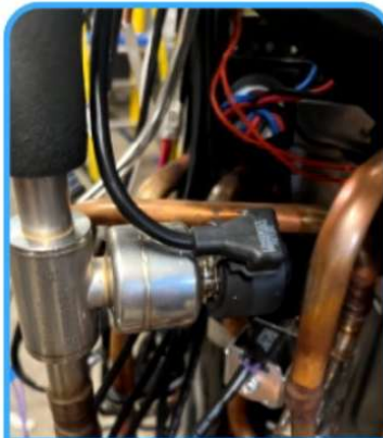
Shutoff valve in multi-zone outdoor units
